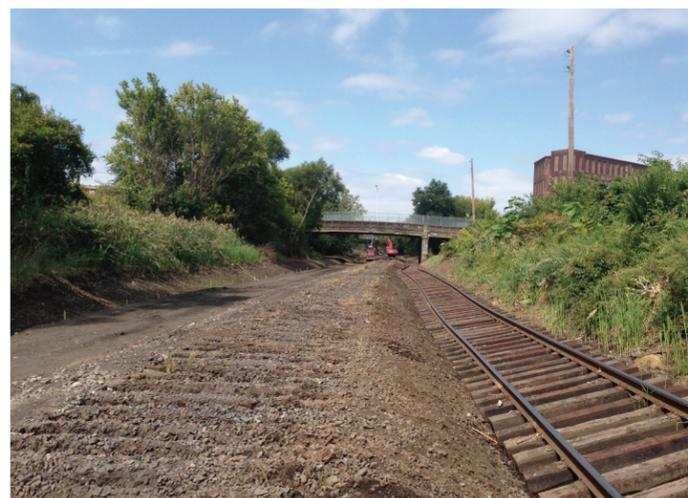
were scheduled. Preliminary projects included advance clearing and grubbing, and the removal of the out-of-service Berks Industrial Track Railroad Bridge. In order to minimize the impact of each outage, ditch excavation and other preparations, including retaining walls, rip-rap ditches and reinforced concrete pipe installation, were done ahead of time, so that the track sections could be removed, excavated and reinstalled quickly in the course of each four-day track outage.
